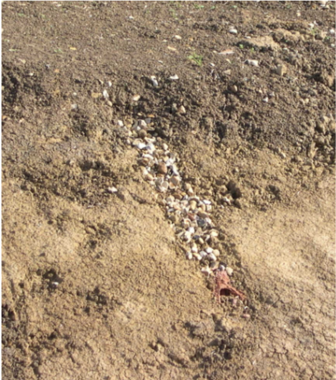
Exposed gravel backfilled clay tile drain
